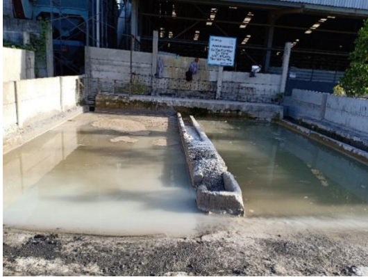
Gambar 1. Kolam Endapan Air Slosch Spun Pile
