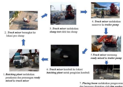
Gambar 2. Proses Operation Pengecoran Plat Lantai
