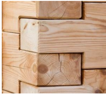
Gambar 2.15. Joint Dove Tail
