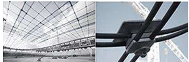
Gambar 2.19. Ilustrasi konstruksi kabel ganda Sumber: http://detail-online.com/article/london-2012-velodrome-16431/
