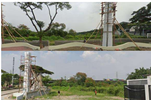
Gambar 1. 5. Lokasi tapak eksisting.
