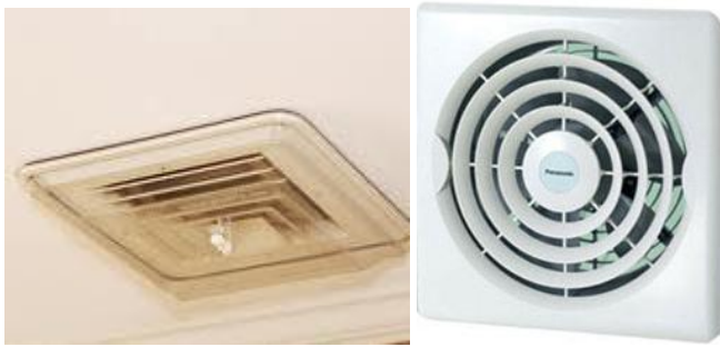
Gambar 4. (a) AC central (b) exhaust fan Sumber: jakartafansupply.indonetwork.co.id
