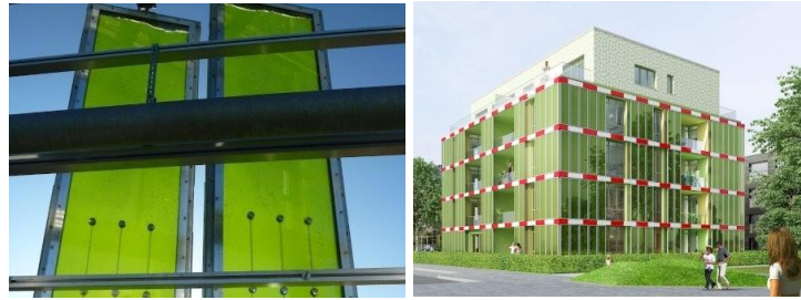
Figure 2. Microalgae facade photo-bioreactor system (Source: https://www.archdaily.com/339451/worlds-first-algae-bioreactor-facade-nears-completion )
